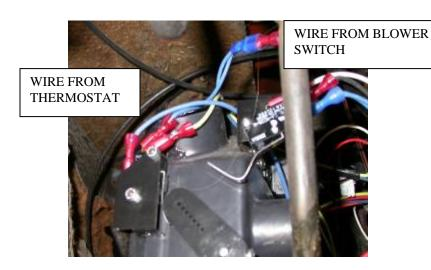
Locate (2) blue wires along the wire harness. Route wires to side of the duct assembly.
